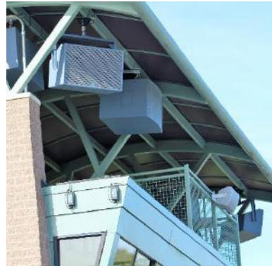
Parkway Sports Stadium Project
