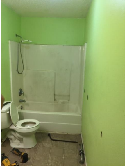
Bathroom Prior to Remodel
